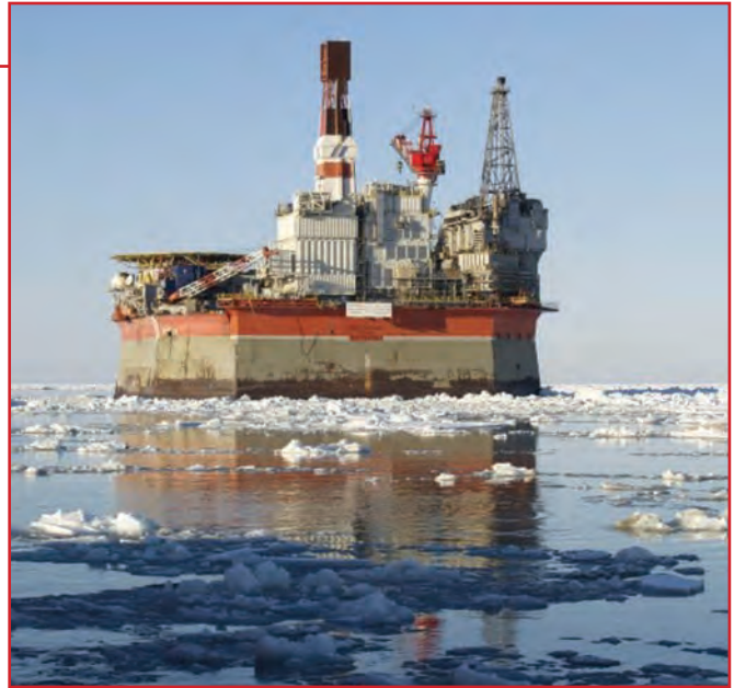
The Molikpaq, a mobile Arctic oil drilling caisson platform designed for operation in the Beaufort Sea
